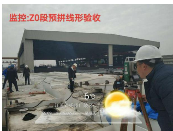
附图 1.0-40 Z0 节段工厂预拼装线形复测
